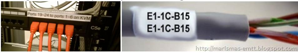
Labeling cables connecting routers/servers/switches during
